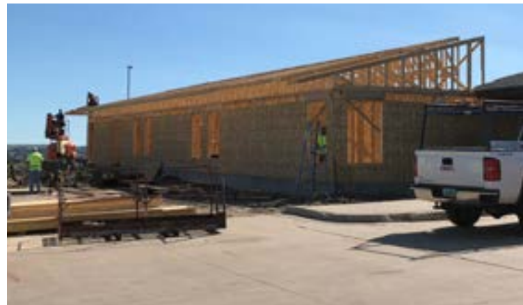
▲ After a vote in February, construction began in April on the expansion. Student Ministry kicked off in the completed wing in December.
